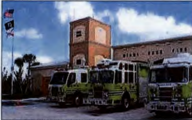
Doral North Fire-Rescue Station 69
