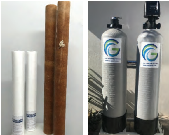
Before & After Filters, from a system installed in Golden Beach
