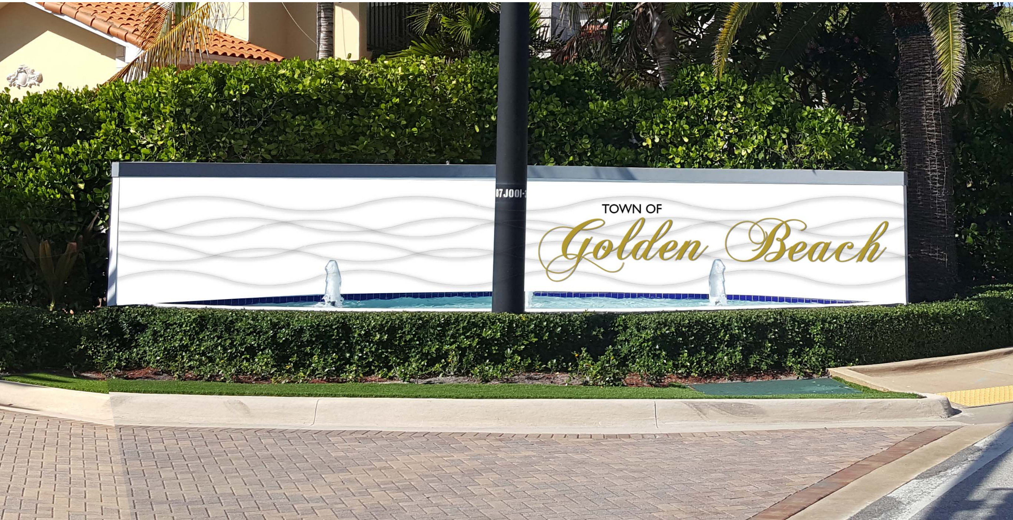
Concept 5: Laser Cut Metal Letters on White Cast Concrete Wall Panels with Wave Motif
